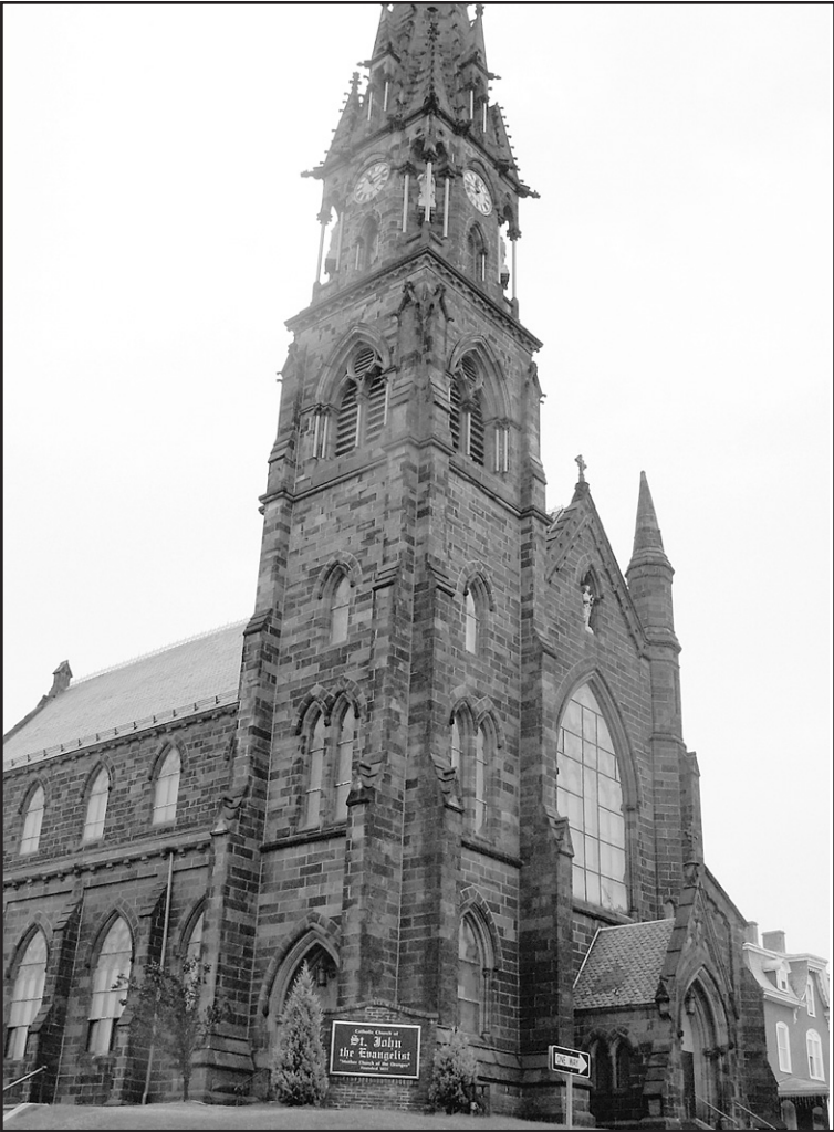
The exterior of St. John's, Gothic in style, and constructed from local brownstone.
