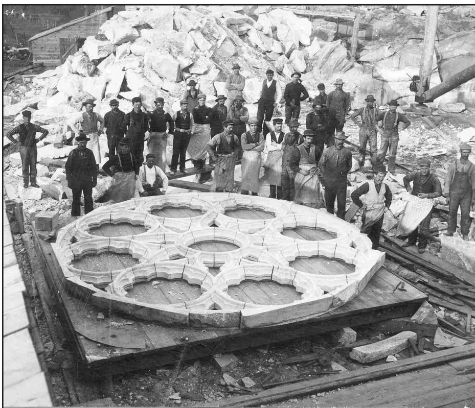
Workers and artisans with the frame for the Rose window during construction of the Cathedral of the Sacred Heart. Photo believed to be in the 1920's.
